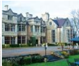
Redworth Hall Hotel Durham, England
